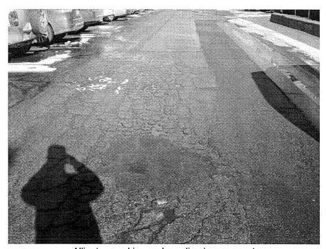
Alligator cracking and ponding in pavement
