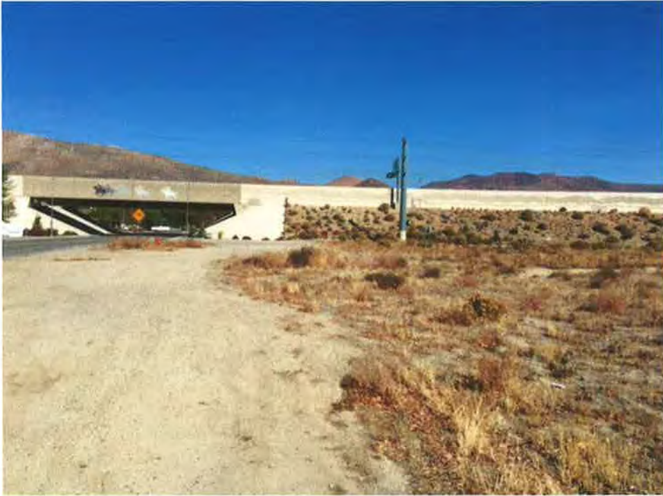
View looking north across property with Emerson Drive on the left
