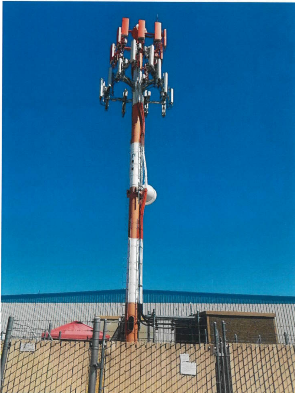
Existing Carson City Airport communications tower. T-Mobile is proposing to collocate an antenna array below the existing panel antennas on this tower.
