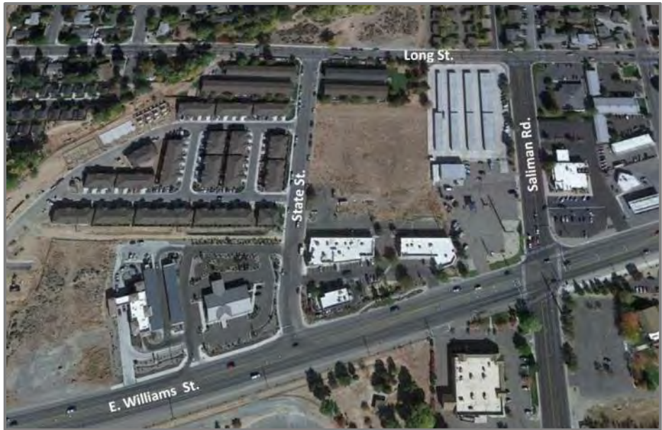
Figure 10: Existing State Street Intersection (Source: Google)
