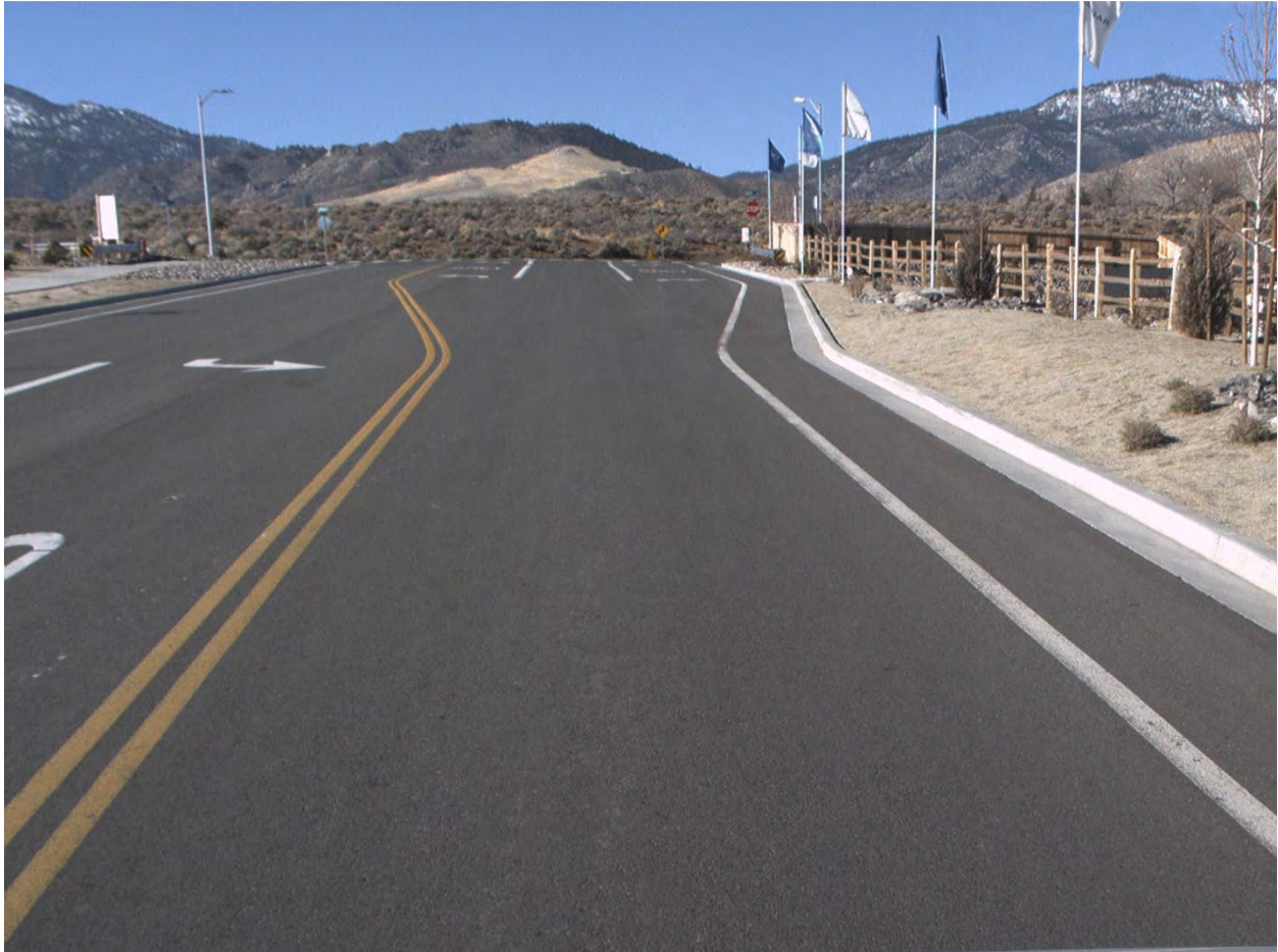
Figure 2. Pavement in Good condition category (PCI 100-86).
